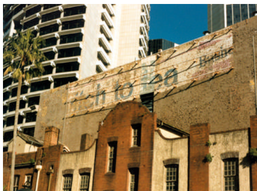
‘Switch to tea’ sign on the northern facade of the Bushells Building before conservation, 1999.
