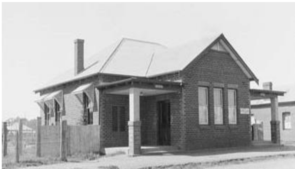
Binnaway Post Office – built 1939-1945 (National Archives)
